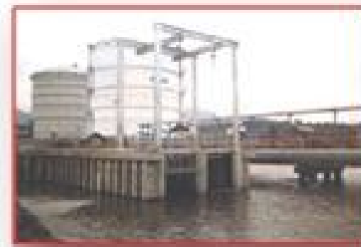
Installation of Lifting System
