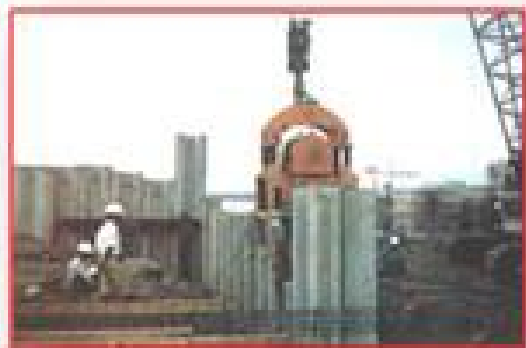
Driving Work with 90 KW Vibro Hammer
